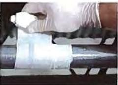
**Tightly wrap** Syntho-Glass, using entire roll, approx. 2" above and below the repair and directly over the rubber tape.
