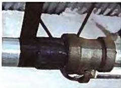
**JOINT:** Cut the provided butyl strip to be sure that it wraps around the entire joint and the ends meet, remove backing and apply. Begin wrapping rubber tape on the outer half and work towards the leaking joint by stretching the tape to its **maximum tension**. Use entire roll of pressure tape and continue to wrap until the leak has stopped.
