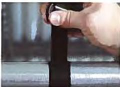
**CRACK:** Use only the rubber tape and be sure that the sealing pad, which has been pre-mounted to the rubber tape, goes directly over the leaking area. Begin wrapping tape by stretching to its maximum tension **DIRECTLY** over the repair area until it has stopped. **DO NOT CHASE THE LEAK** as each wrap provides additional pressure over the leak.
