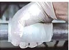
**Squeeze and mold** Syntho-Glass in the direction of wrap, removing excess water and spreading resin until tacky to touch (approx. 3 min.). Wait 30 min. at 75°F before returning to operating pressure.
